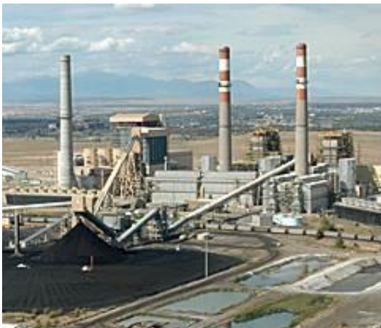
Commanche Generating Station, near Pueblo At 1426 MW, the largest power plant in Colorado It burns Wyoming coal in 3 units and is operated by Xcel Energy
