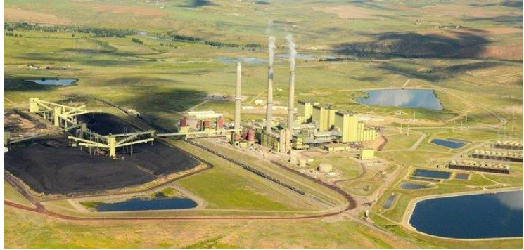
Craig Generating Station
