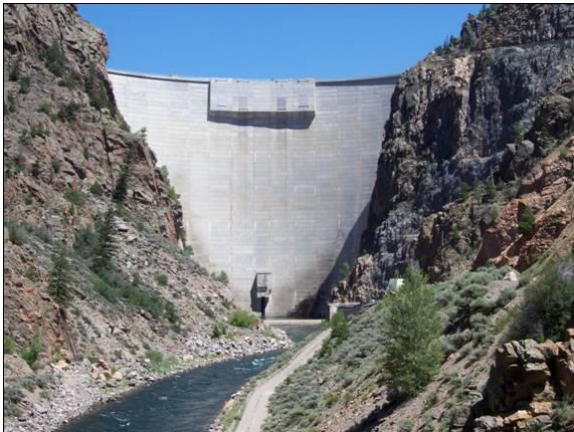
Morrow Point Dam & Power Plant U.S. Bureau of Reclamation Cimarron, Colorado
