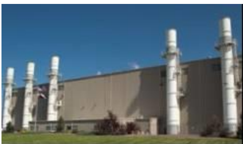
J. M. Shafer Generating Station in Fort Lupton Natural gas fuel. Combined cycle operation. 272 MW from 5 units. Owned by Tri-State.
