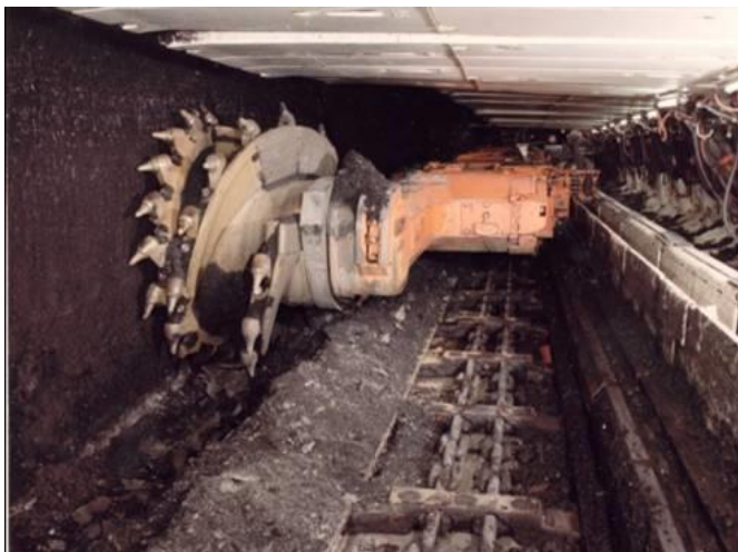
A coal shearer in action. Shields above and to the right. Conveyor below.
